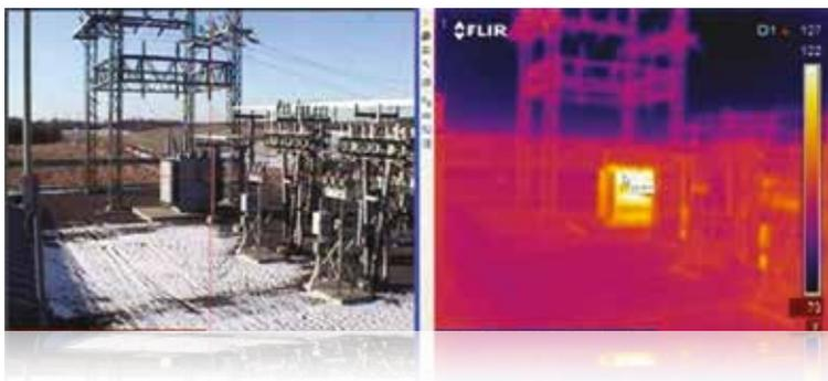
The cameras can be installed on a pan/tilt mounting mechanism to continually survey large areas of a substation. A few cameras can provide real-time coverage of all the critical equipment that should be monitored. In addition to preventative maintenance functions, these cameras also serve as security monitors for intrusion detection around the clock.
